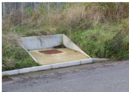
Poorly integrated drain cover on Iseham Road
